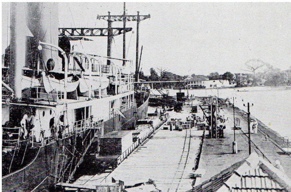
Conakry. — Le wharf
