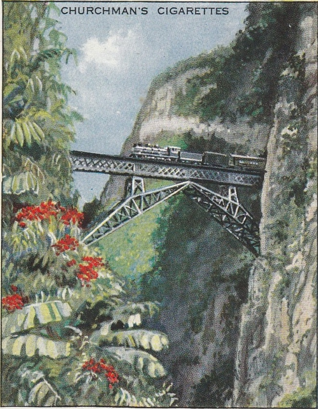
FAUX-NAM-TI BRIDGE, INDO-CHINA
